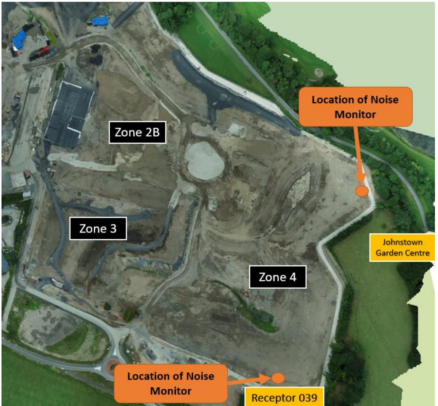
Figure 8-3 Earthworks in Zone 2B & 4. Nearest Receptor 039
