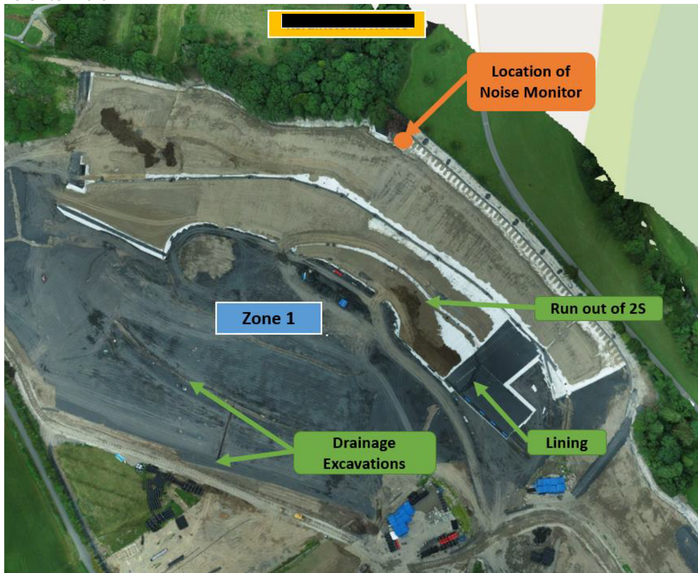
Figure 8-1 Earthworks in Zone 1. Nearest Receptor 001
