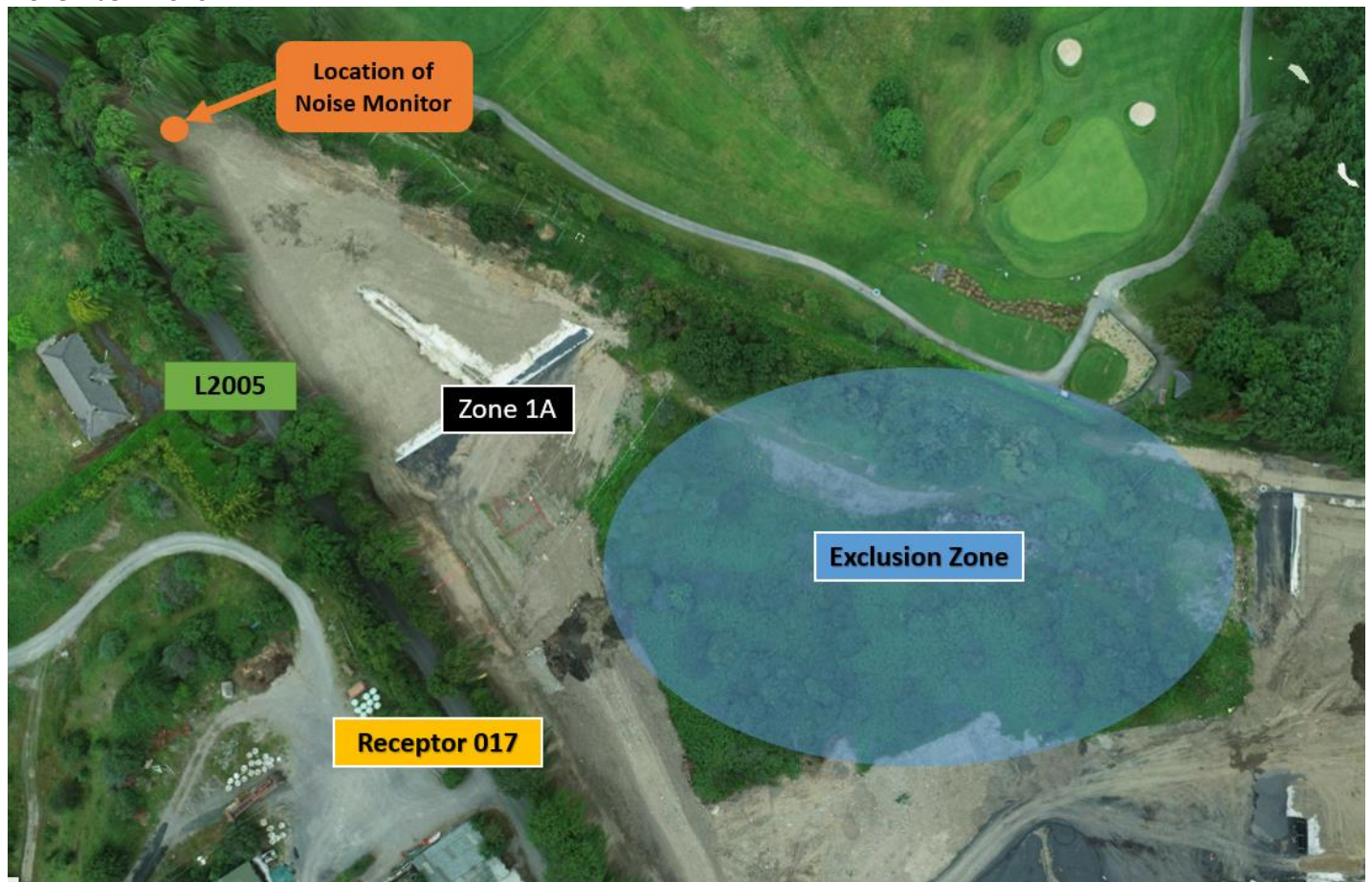
Figure 8-2 Earthworks in Zone 1A. Nearest Receptor 017
